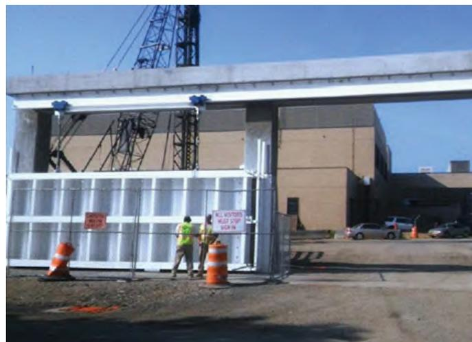
*Figure 6: Over-head trolley roller gate at Bay Park Wastewater Treatment Plant. (Source: Arcadis)*
