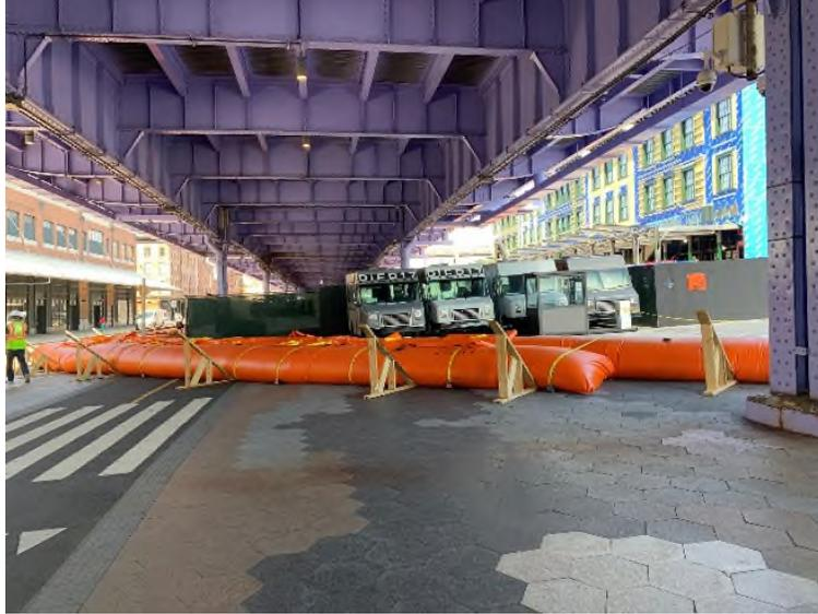
Figure 2: Temporary water-filled tubes (Tiger Dams) in Lower Manhattan. (Source: NYCEM)
