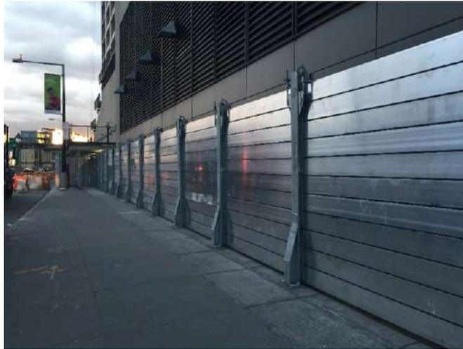
Figure 4: Plank-type system installed at (Source: NYCEM)
